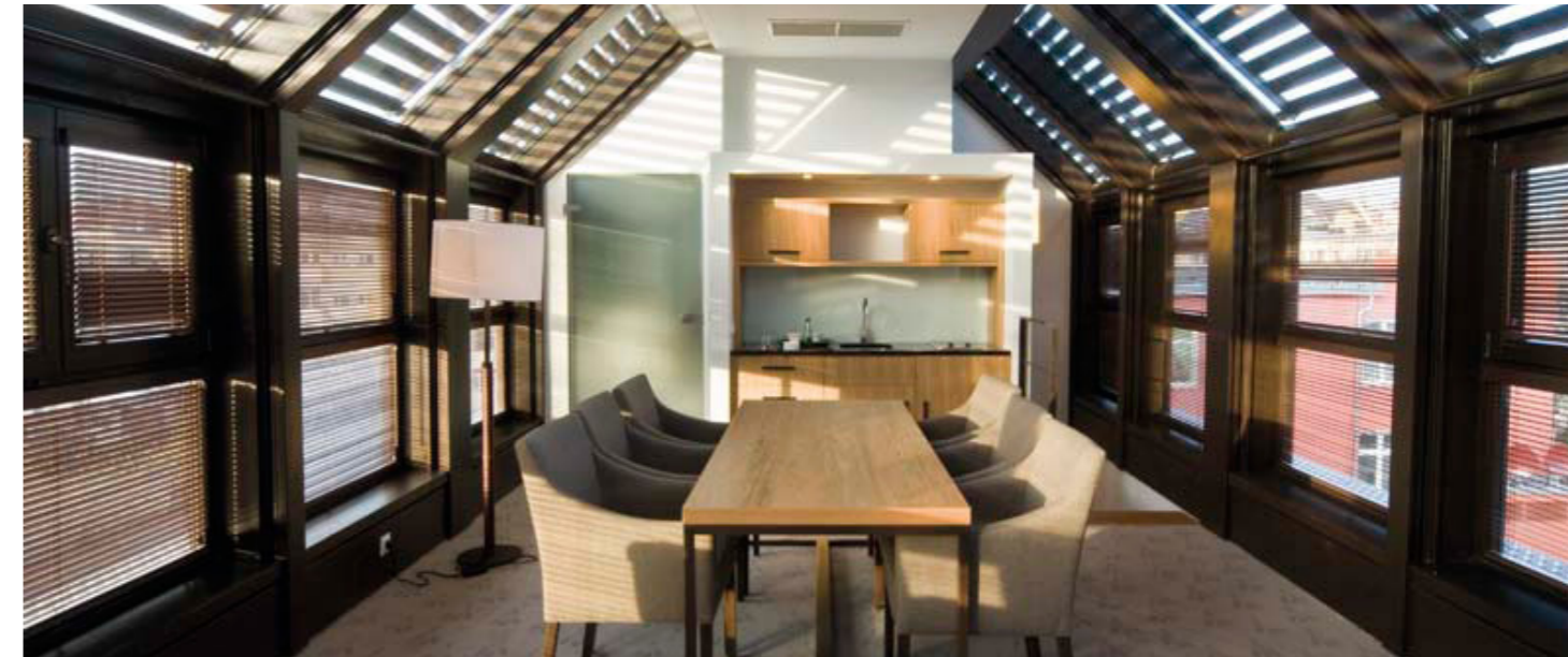
Dining room with adjoining kitchen on a glazed mezzanine. Oak elements fastened to frames made of raw steel covered with imitation rust.
